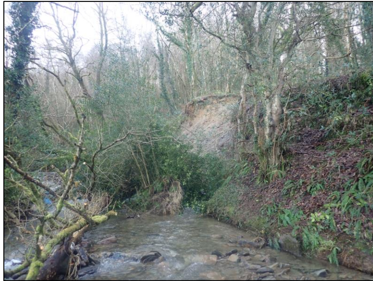
Figure 26: Photo of localised landslip on the embankment of the Nant Cae Dudwg watercourse (image captured by RCT's Flood Risk Management team on 02/03/2020)
