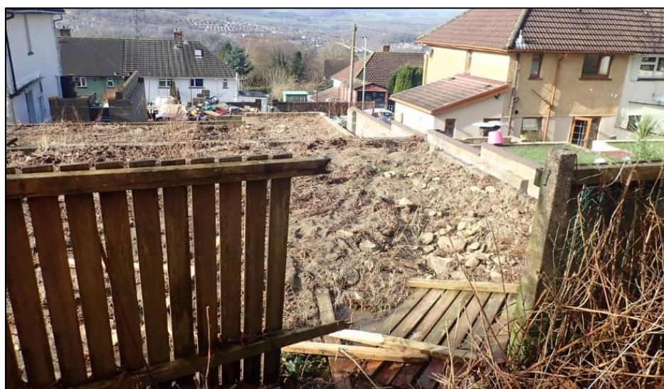
Figure 9: Damages to rear garden of a property at Heol Mynydd following the storm event (captured by FRM officers on 17 th February 2020)
