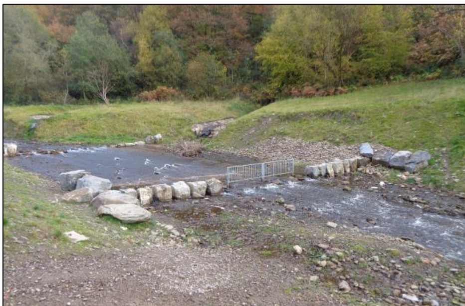
Figure 24: Initial upstream debris screen in the Nant Cae Dudwg watercourse captured prior to Storm Dennis
