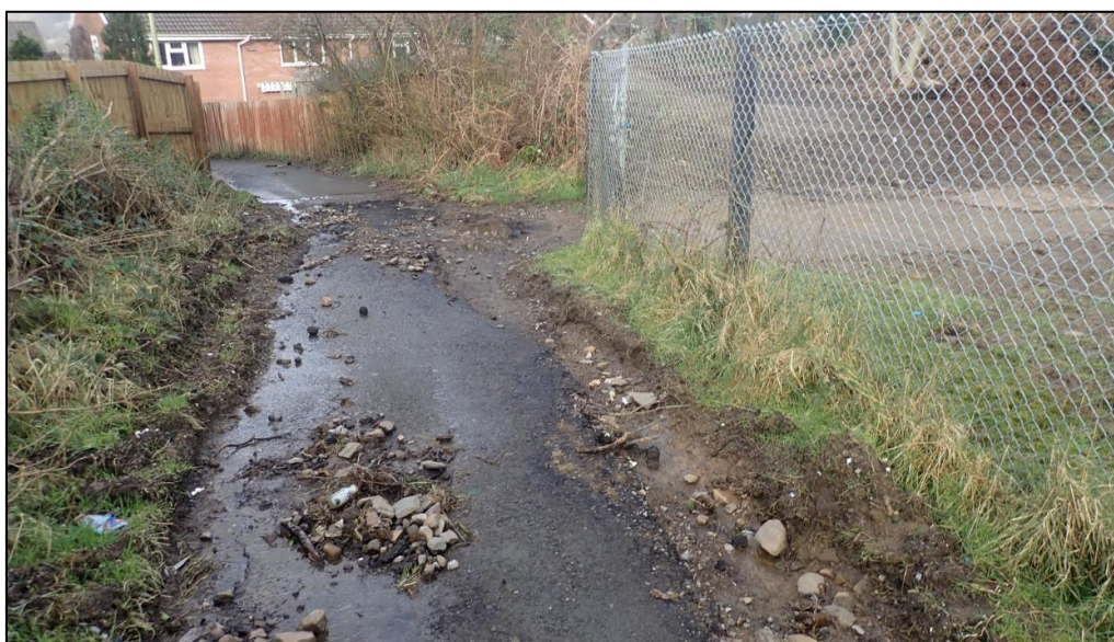
Figure 12: Evidence of deposited debris and damages to the bottom of the path looking down towards Brynderwen. Overland flows were observed flowing through land to the right behind the fencing (captured by FRM officers on 17 th February 2020).
